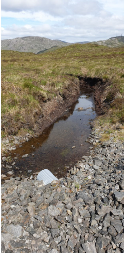
Plate 9.2: Example of Track Culvert Discharging to Enhanced / Cut Drainage Channel
