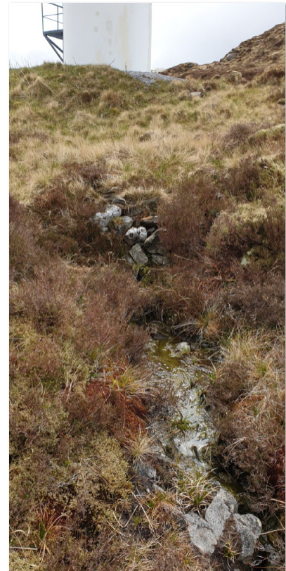
Plate 9.4: Example Drainage Discharge Point and Channel Associated with Existing Turbine Foundation
