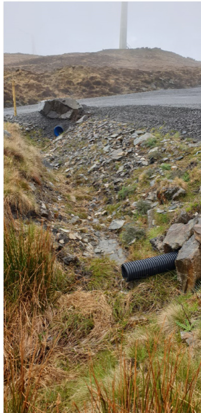
Plate 9.3: Example of Track Culverts and Drainage Channel Adjacent to Existing Track
